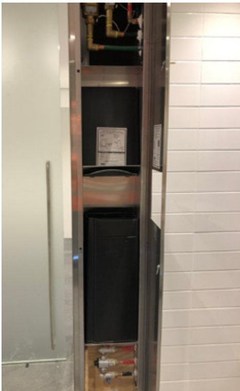
Bobrick's B-38033 TrimLineSeries™ Recessed Paper Towel Dispenser, Automatic Hand Dryer and Waste Bin was customised for use in 6&8 Parramatta Square to fit a tight space that also had to accommodate plumbing.
